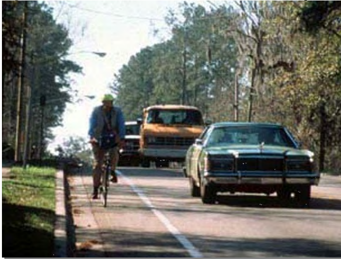
Figure 5 Bike Lanes with a Curb and Gutter System
