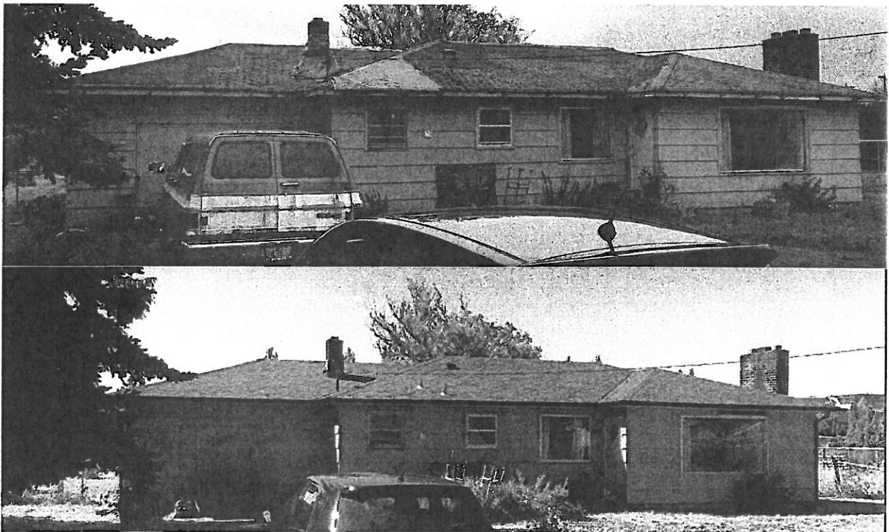
Above: Before and After where a homeowner in unincorporated Marion County received a new roof and repairs to interior drywall resulting from previous leaks from the damaged roof.
