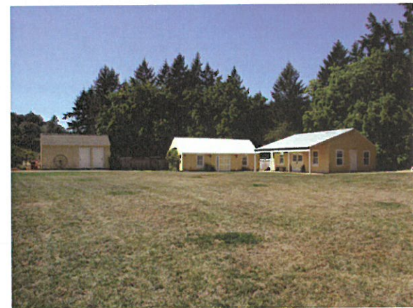
Well House, Commercial Kitchen, and Museum
