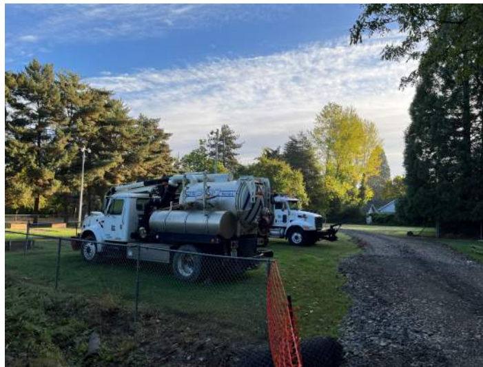
Figure 2 Staged equipment – vac truck, dump truck, excavator (between trucks).
