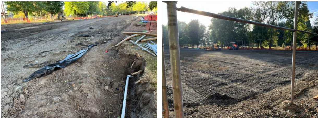
Figure 1 Base aggregate and fabric – Currently being placed, graded, and compacted.
